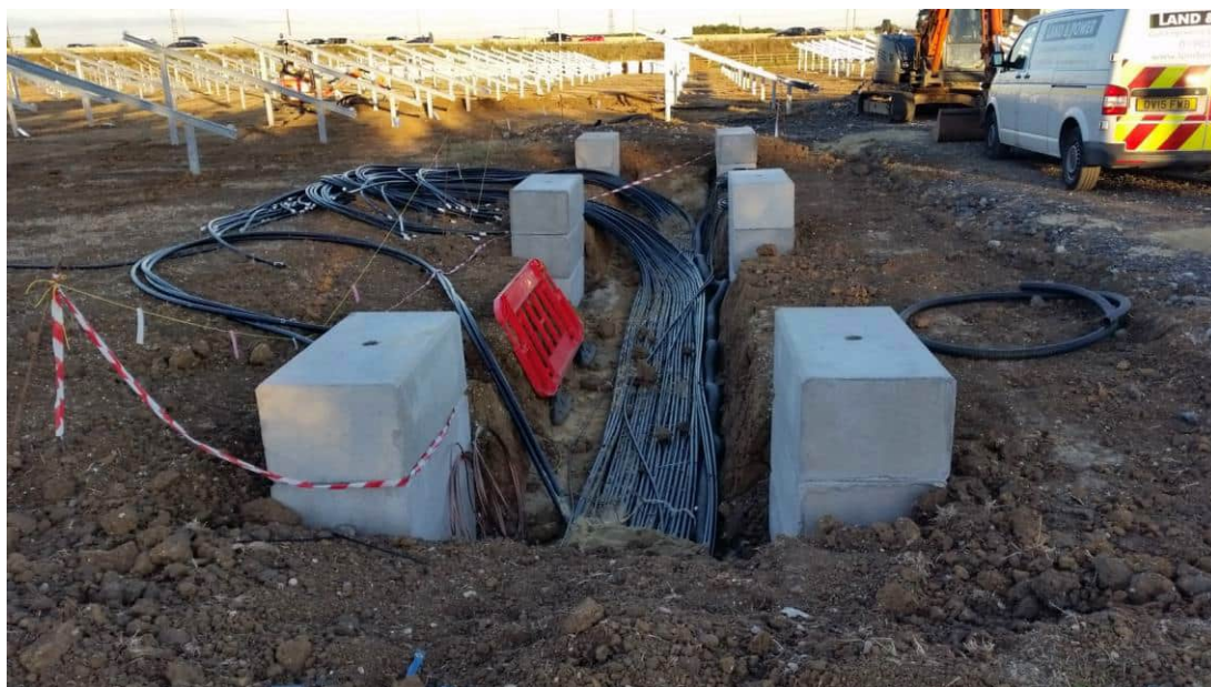
Plate 2-8: Example Underground Cable Installation
